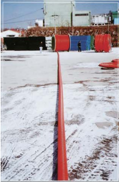
▲ Demonstration of straightend COD
