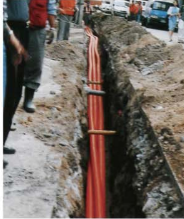
▲ Laying of COD through/under hurdles.
