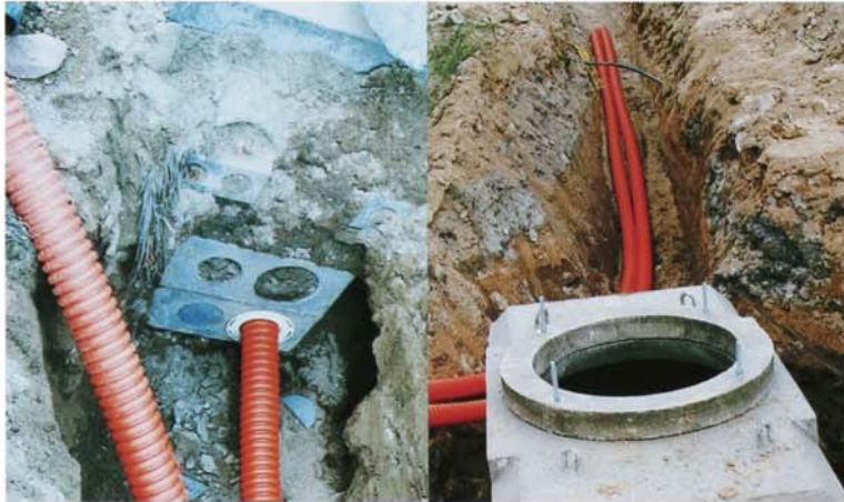
▲ Multiple COD line installation work for 500m mahole interval.
