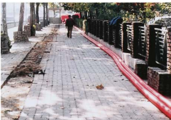
▲ Temporary COD laying along walkway.
