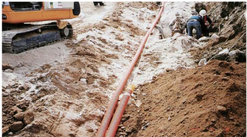
▲ COD laying out of 400m long customized roll.
